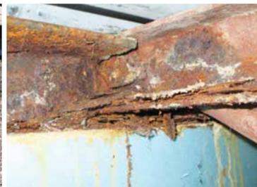
Rusted building structure steel in the crawlspace of a school.
