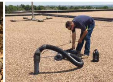
Smoke tests are done to find failing sewer lines in need of repair.
